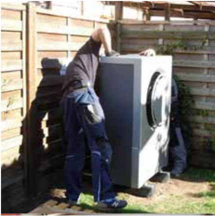
Thermia Atec during installation
