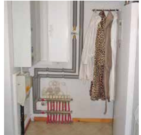
Thermia Atec indoor unit and manifold for heat distribution
